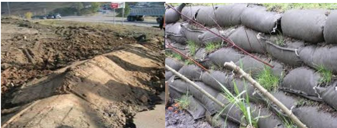
Fig:3 Heap earth barriers and Sandbags fill barriers.
